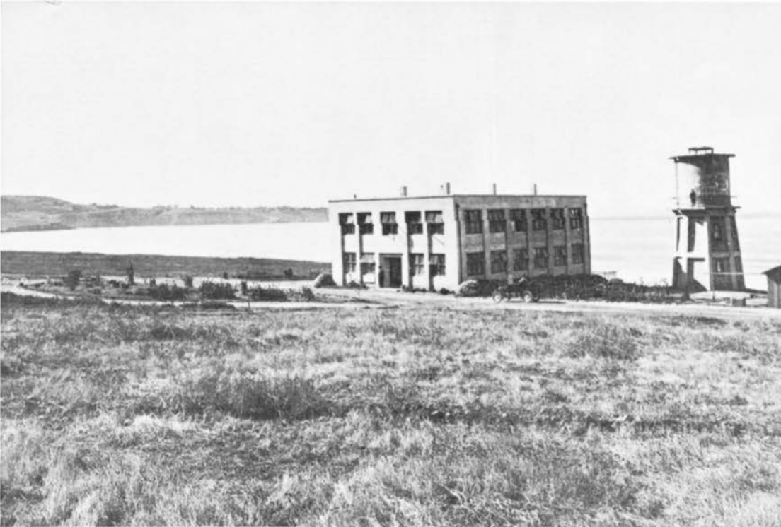
George H. Scripps building just completed in 1910, still in use in 1966.
