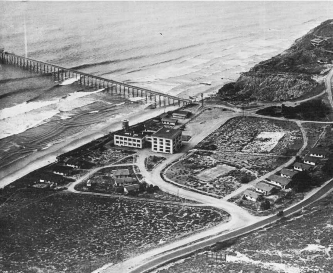
The Scripps Building, (center left, above) became the nucleus of a complex of buildings which by 1916 included the museum library (joined to the Scripps Building by a bridge), the aquarium (behind the two larger buildings above), the pier, the Director's home (on the triangle of land, above right) and housing for visitors and staff scattered over the hillside.
